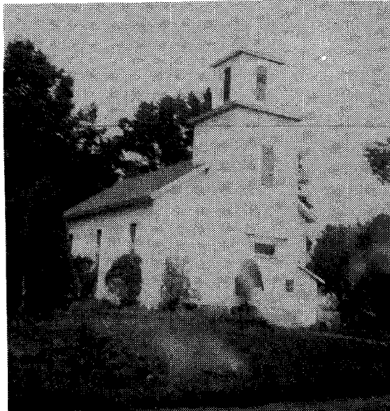
Building prior to new entryway
